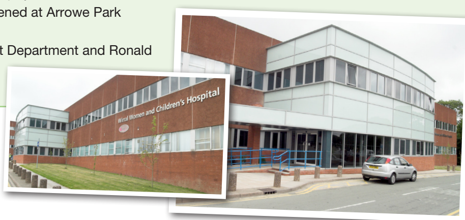
NEW LOOK: The newly completed entrance to our Wirral Women and Children's Hospital.
